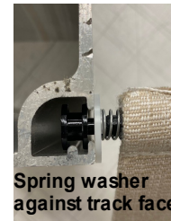
Wheel guide & wheel in correct position
